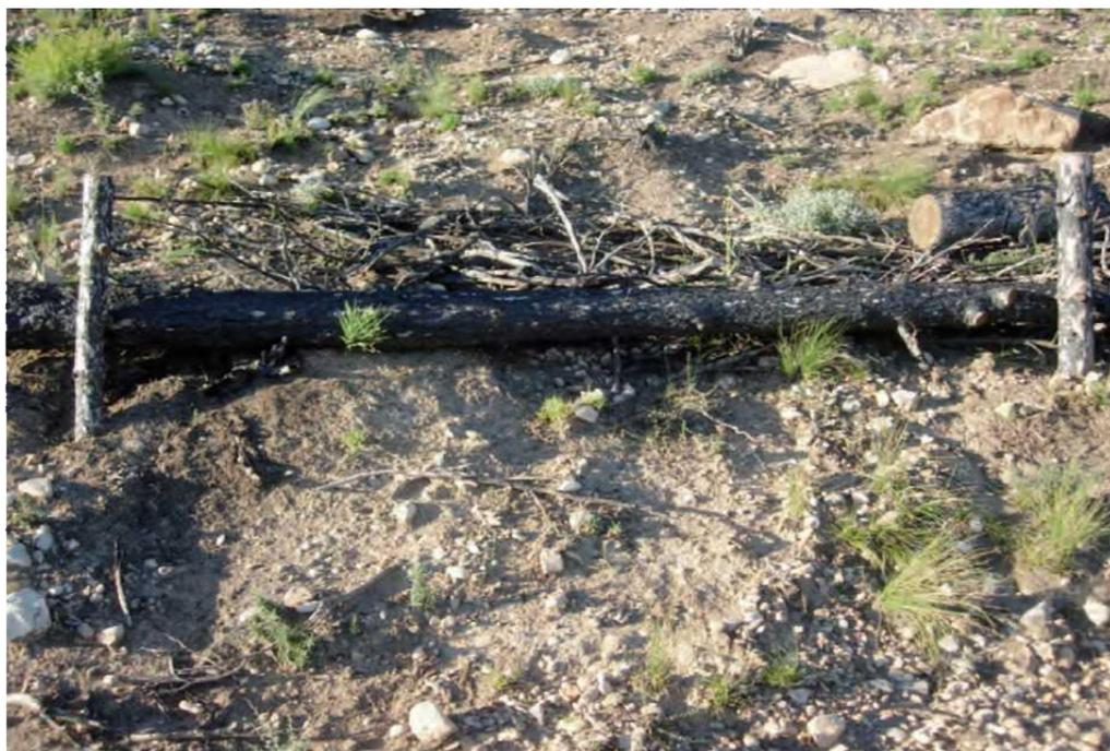
Figure 3. Erosion barrier
